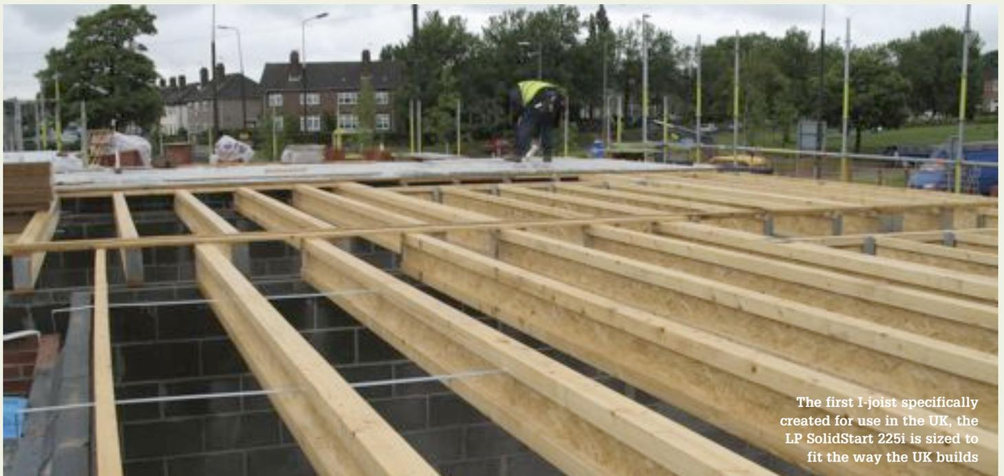
The first I-joist specifically created for use in the UK, the LP SolidStart 225i is sized to fit the way the UK builds
