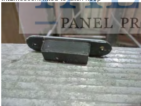
Intumescent fitted to latch keep
