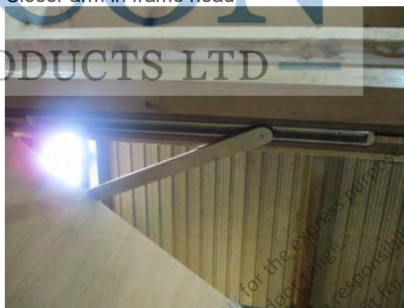
Closer arm in frame head
