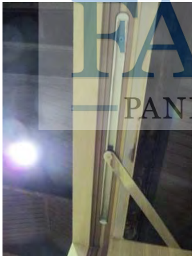
Closer arm channel in frame head
